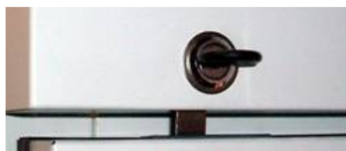
Detail of door lock
